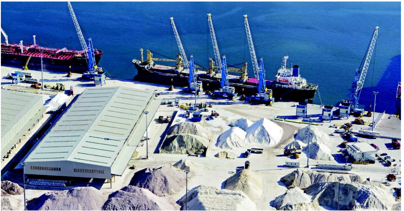
North Terminal at the Ravenna port, in Italy Il terminal Nord a Ravenna
